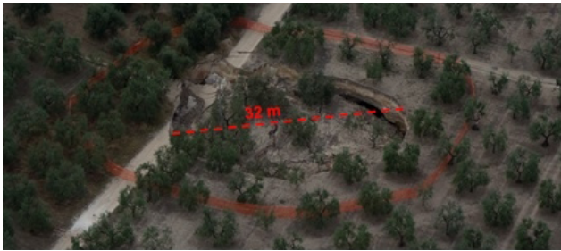
Figure 5. Aerial view of the sinkhole that occurred in the Barletta area.
